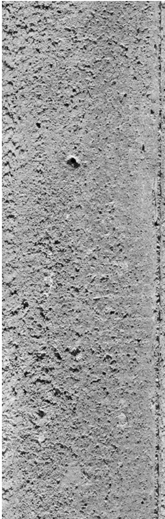
Reinforced concrete walls
